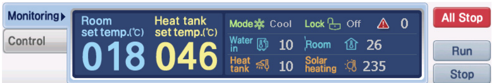
<AWHP unit monitoring tab - When control temperature is set to air temperature >
