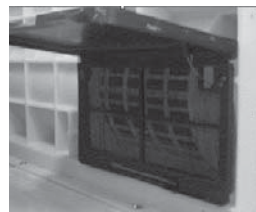
Figure B – Vent Filter Removal
