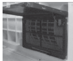
Figure B – Vent Filter Removal
